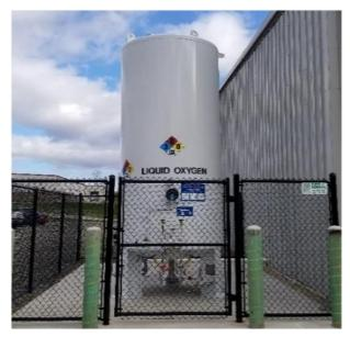
One method to reduce the likelihood of a fire is to separate the oxygen source from other exposures. National Fire Protection Association 55, Compressed Gases and Cryogenic Fluids Code includes the following table of exposures and recommended separation distances.
